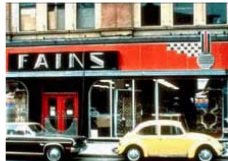
This 1930s Moderne storefront has gained significance over time and should be preserved. Photo: NPS files.
