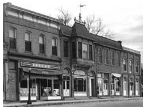
By evaluating the components of a storefront as well as their existing condition, a successful rehabilitation is more likely. Photo: HABS collection, NPS.
