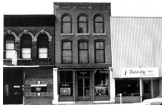
This photograph shows the impact of preserving historic storefronts. The one on the right has been totally obscured by a "modern" front added in the 1950s. Photo: NPS files.
