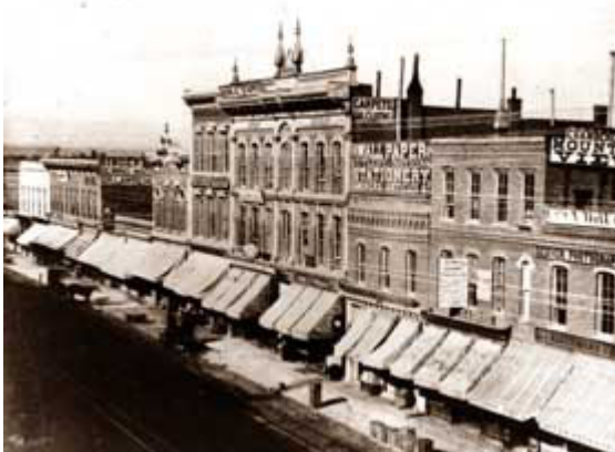
Try to locate old photographs or prints to determine what alterations have been made to the storefront and when they were undertaken. Awnings were common elements of storefronts at the turn of the century. Photo: NPS files.
